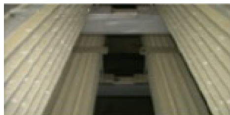
Fig 7c: Salt can be seen forming on the aluminium extrusion. These extrusions are shown supported and strapped to the structural stainless-steel box-section.
