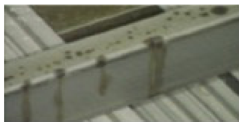
Figure 7a: Corrosion is seen forming here, predominantly on the central weld of an LDX 2101 stainless steel box-section. Corrosion product is visibly dripping down onto the underlying (finned) aluminium extrusion.
